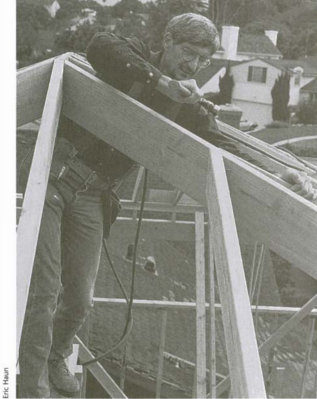
With the hip rafter in place, the jack rafters can be nailed on, beginning with the longest one.
