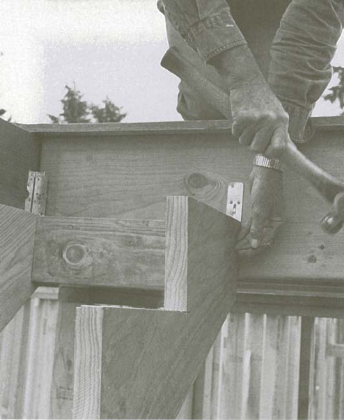
Stair stringers need to be fastened securely to the header joist.
