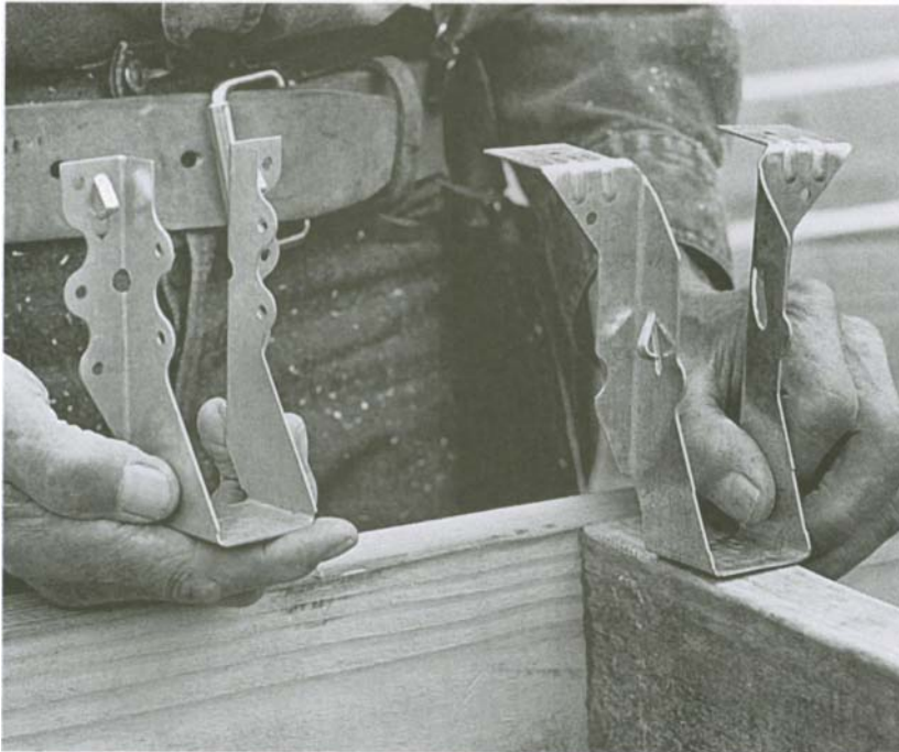
The joist hanger on the right hooks over the supporting beam or joist and requires fewer nails to install than the hanger on the left.
