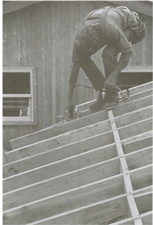
To ensure a straight fascia, mark and cut the rafter tails to length after the roof is stacked.
