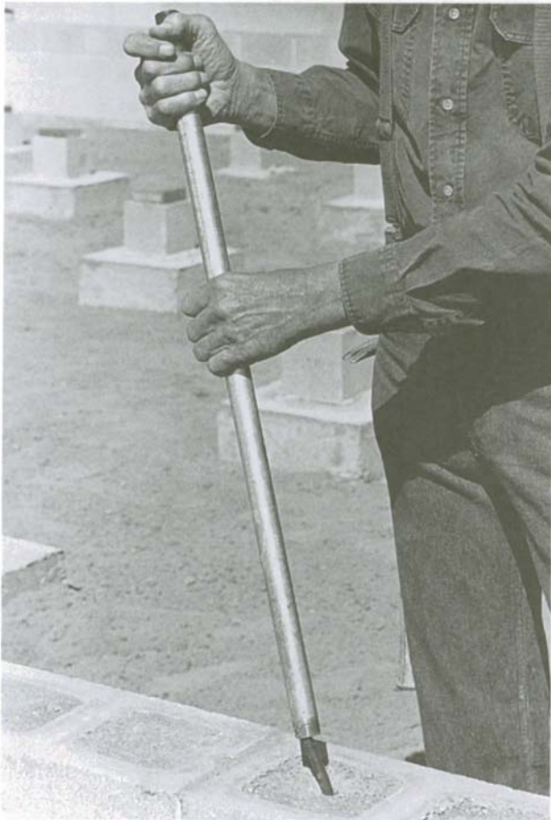
Bent anchor bolts can be straightened easily with a piece of 3/4-in. pipe.
