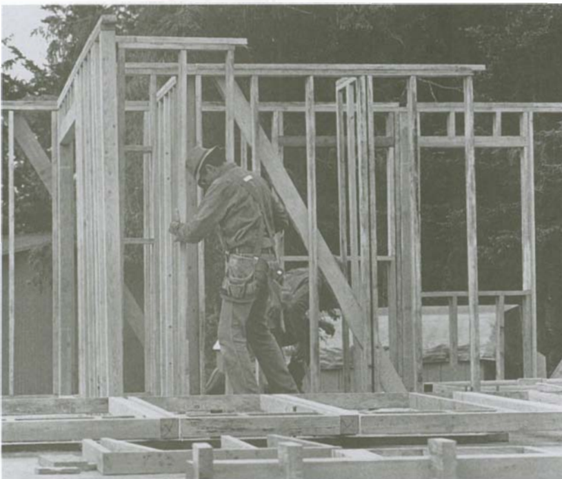
Intersecting walls are raised and tied into other walls.
