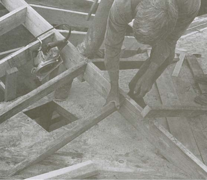
The blind-valley jack rafters are nailed from the ridge to the 1x base, which is secured to the main roof.
