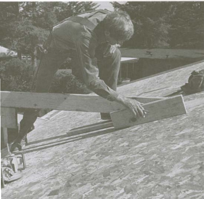
Top: The blind-valley ridge can be marked to length by extending a second piece of ridge to the main roof. Above left: Lay another piece of ridge stock alongside the extension on the main roof and scribe the pitch of the roof on the extension. Above right: Cut along the pitchline and the extension can be nailed in place.
