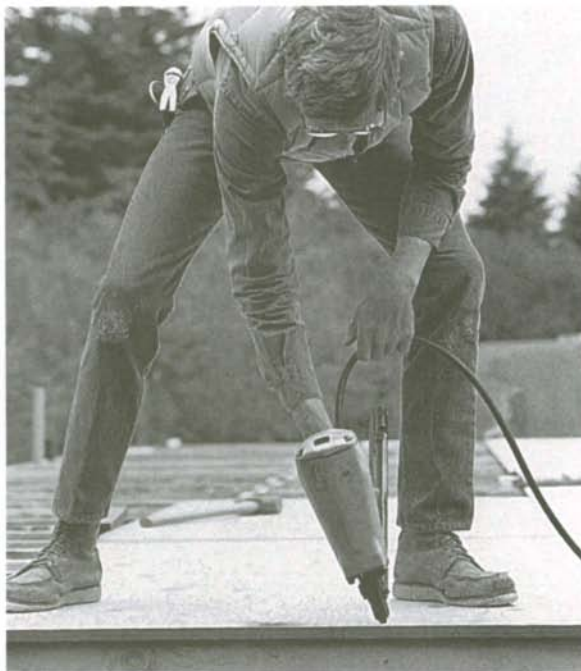
Pneumatic nailers make it easy to nail down floor sheathing.
