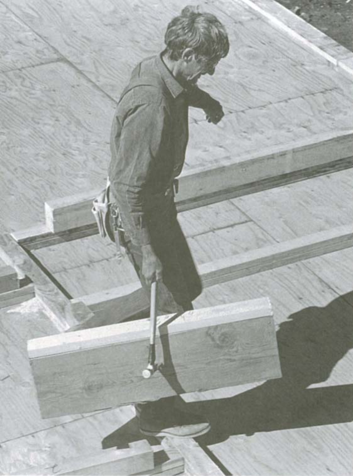
Picking up and carrying headers with a straight-claw hammer can save wear and tear on your back.
