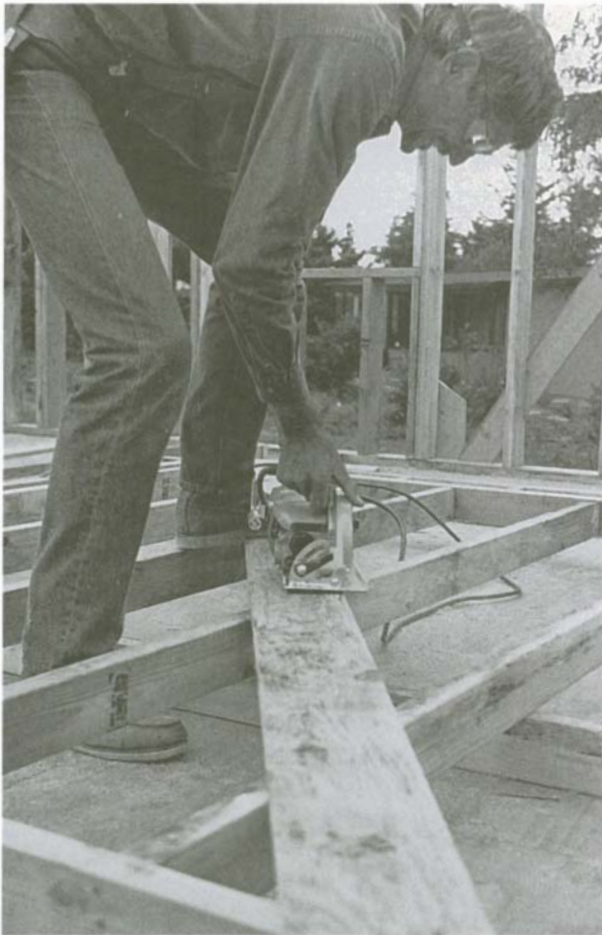
To cut out studs for a 1x let-in brace, lay the brace stock along the wall in its intended location. Using the brace as a guide for your saw, cut along both sides.
