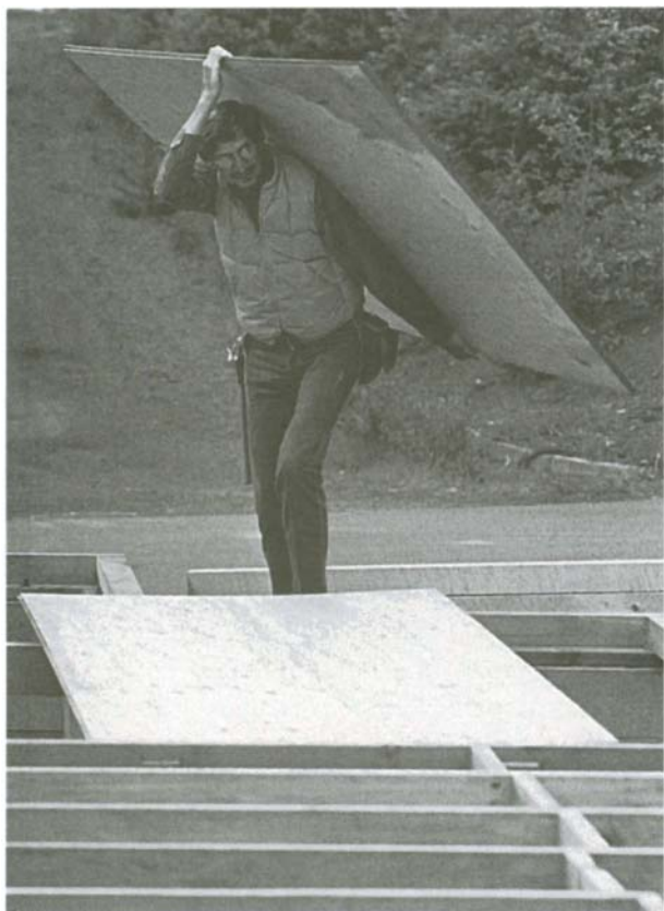
Sheathing panels should be carried with one hand on top and one on the bottom, with most of the weight resting on the shoulder.
