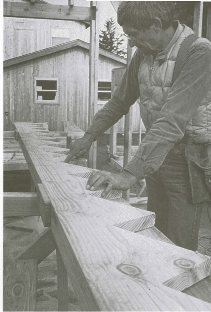
Once the first stringer is cut, it can be used as a template to mark the others.
