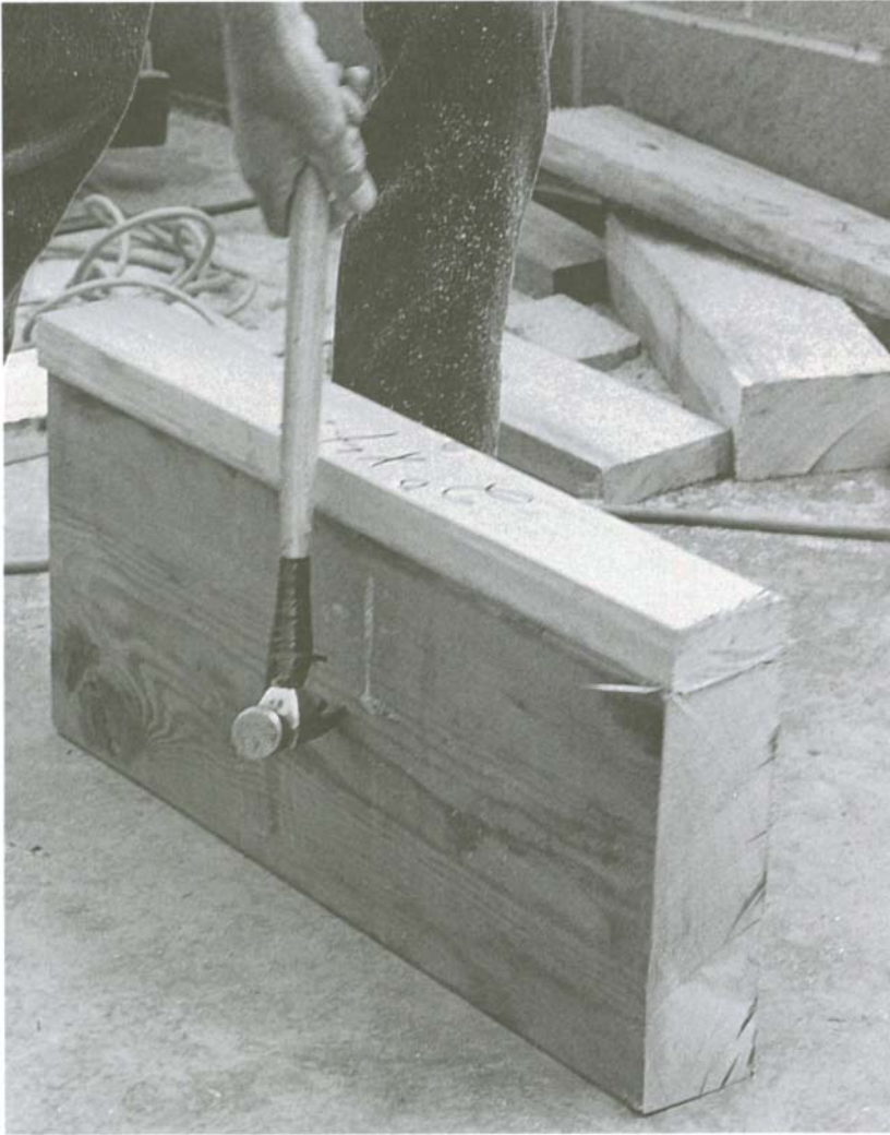
Solid-stock headers like this 4x12 can be nailed directly to the top plate, thereby eliminating all top cripples.
