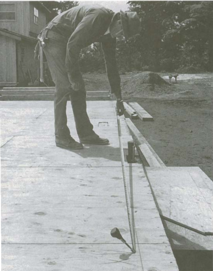
An efficient framer will make good use of an awl on a layout job. Stuck in the subfloor, it can hold one end of a chalkline or measuring tape.
