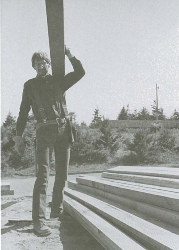
A 16-ft. long 2x6 can be heavy. Learn how to carry sill stock on your shoulder.
