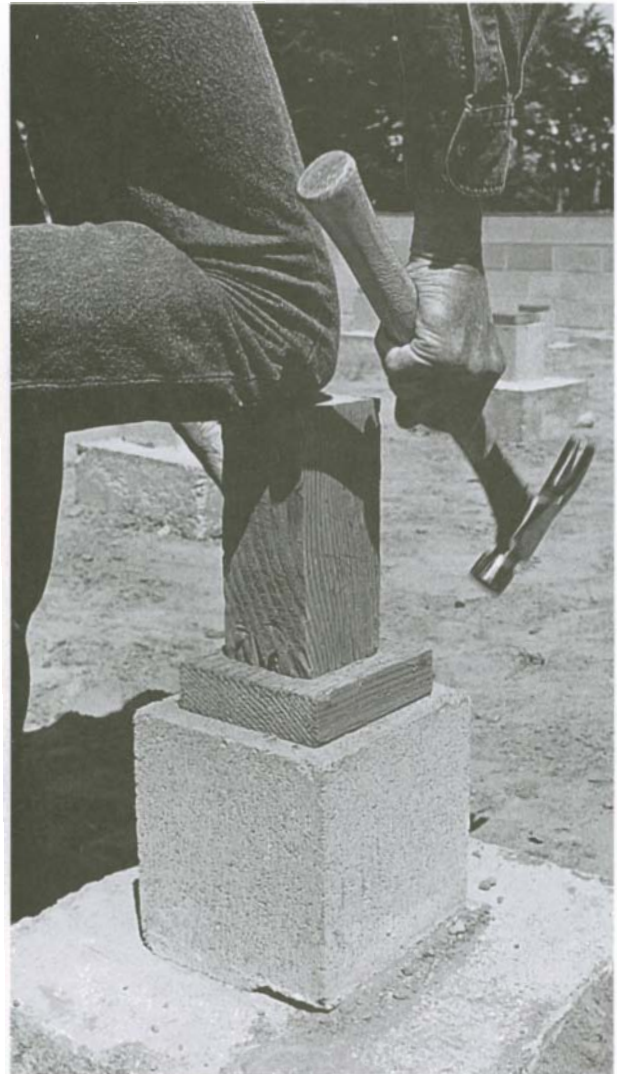
Each post is nailed to the pier block with three 16d or four 8d nails.
