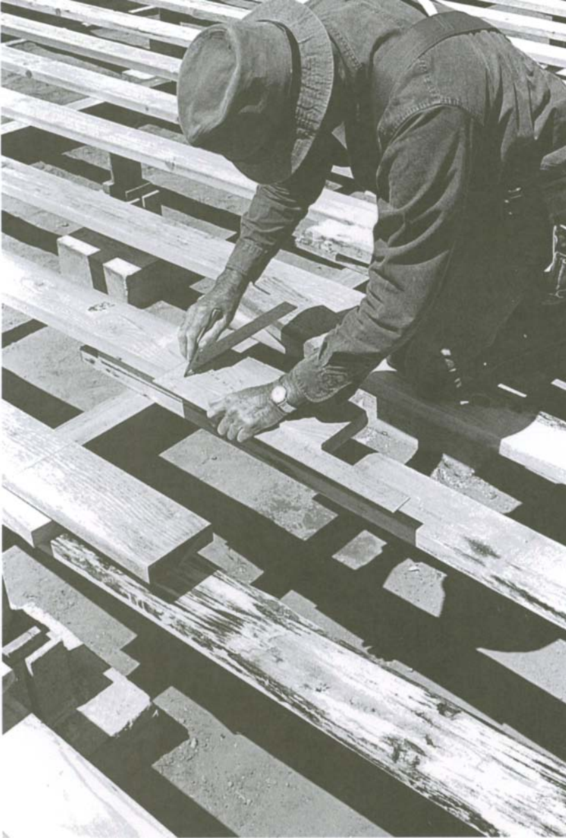
Blocks can be marked to length quickly using a framing square.
