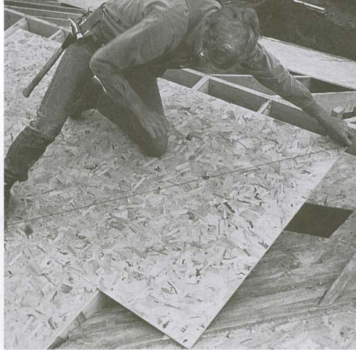
3. Connect this point to the upper corner with a chalkline.
