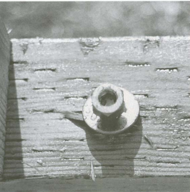
Exterior walls on a concrete slab are secured with nuts tightened on the bolts.
